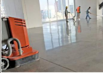
All WerkMaster machines edge to within 1/8" (3 mm) of the wall. No further edge work is required.
